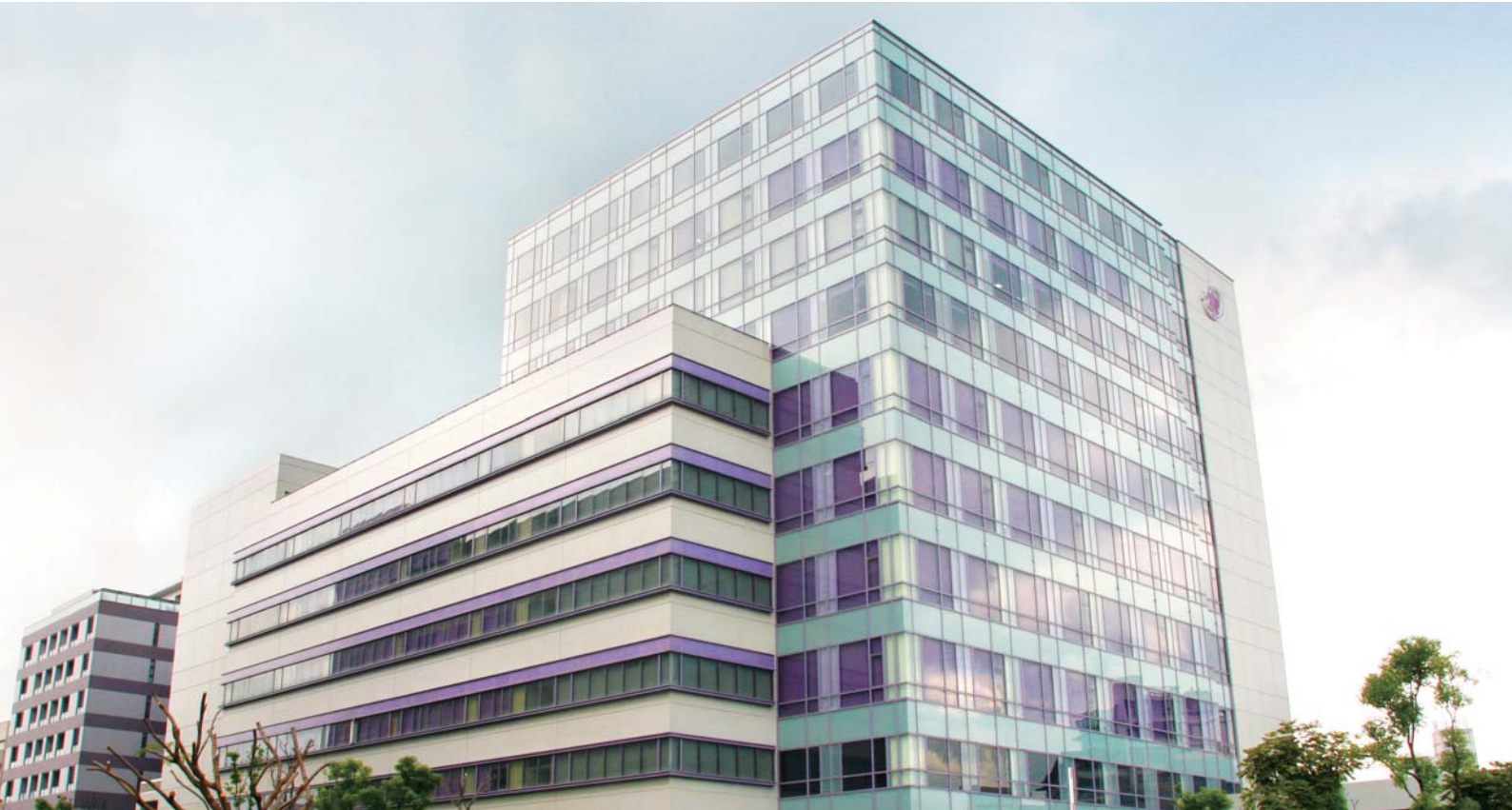
Portwell Engine (PE) Building
